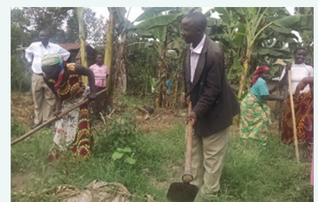
Ground breaking for piggery project
